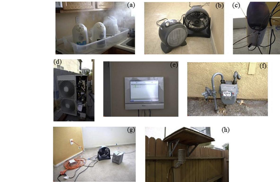
**Fig. 4.** (a–h) Building systems and sensors including: (a) humidifier, (b) electric heater and fan, (c) temperature and humidity sensor in a guest bedroom, (d) VRF outdoor unit, (e) intelligent control system, (f) smart meter for the whole house, (g) electricity monitoring for the electric heater and fan, and (h) the weather station.
