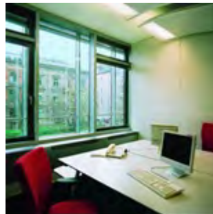
Fig 5. Offices with operable windows and sun protection, allowing natural ventilation and lighting.
