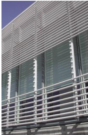
Figure 1. Example of high performance façade used on the New York Times HQ tower in NYC. Consists of “layered” design solutions, A) inside-to-outside and B) floor-to-ceiling. A) consists of 1) External fixed ceramic rods for shading for solar control and daylight diffusion; 2) High performance insulating glass unit with spectrally selective low-E coating, argon gas fill and low-iron glass, including some fritted sections for glare control; 3) Interior automated, motorized roller shade with shade material selected to balance daylight admission and glare control. B) consists of 1) plenum and upper glazing zone for glare control and light diffusion; 2) central unobstructed vision area; 3) lower partially shaded zone that admits daylight to bounce off the unoccupied floor area adjacent to window. ( Lee et al, 2005)
