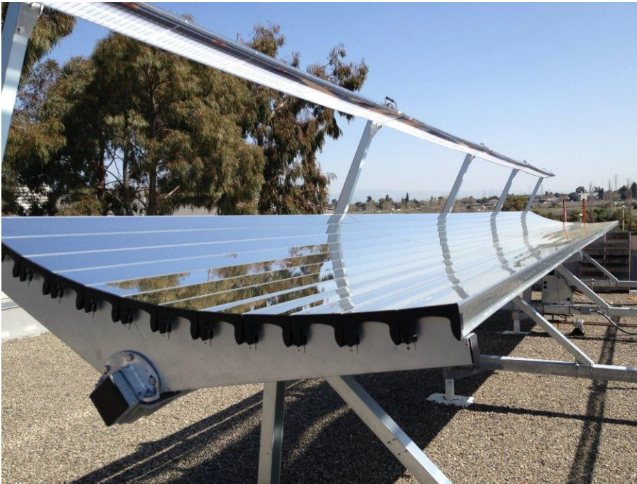
Figure 3. 44-module solar cogeneration system on the roof of one of the cafes. The system has a capacity of 106 kW thermal and 20 kW electrical and will substantially offset the energy required to produce hot water for the cafe.
