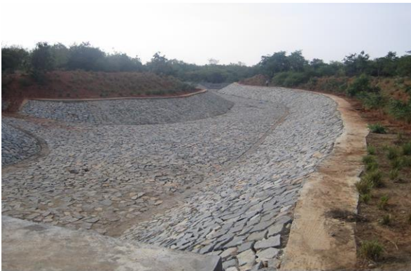
Figure 6. Earthworks for the water management system under construction.
