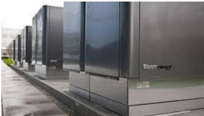
Figure 2: Adobe has installed 12 100 kW Fuel Cells by Bloom Energy on its 5th floor parking garage.
