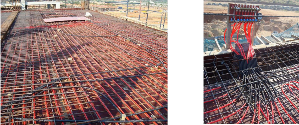
Figure 1. Radiant slab tubing, prior to concrete being poured (Photo courtesy of Infosys Limited)
