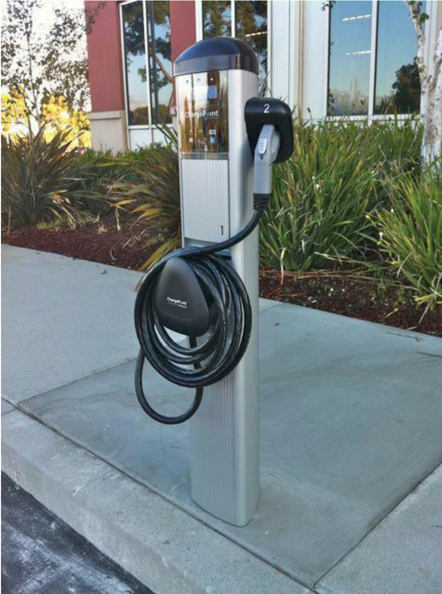
Figure 4. One of 25 electric vehicle charging stations.
